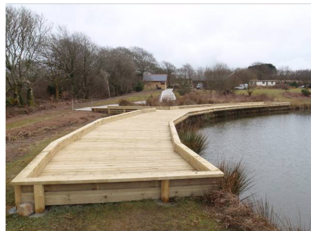
Angling platform specifically designed for tuition.
